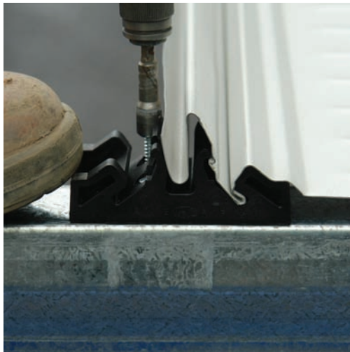
(c) RT-block being secured to Thermo-bar Plus
