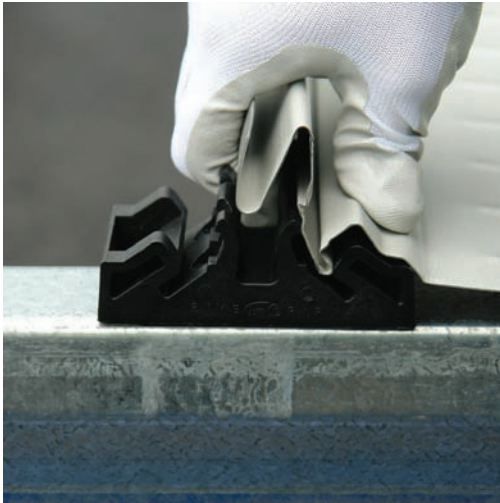
(a) Underlap of sheet being clipped into RT-block
